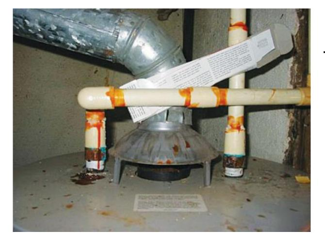
CPVC pipe touching the flue pipe? The fix? Slip some card board between the warm flue pipe and meltable plastic!
